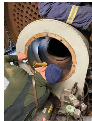
CWO Mike Mitchell inspecting the fireside internal of a boiler.
